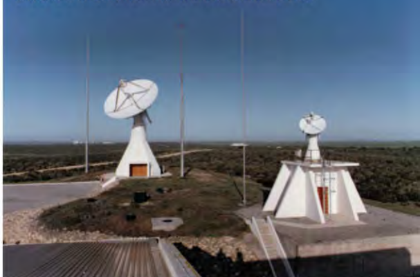
GROUND STATION CONTROL ROOM
