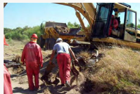
■ The area was cleaned and the soil sieved to ensure that the area was clean.
